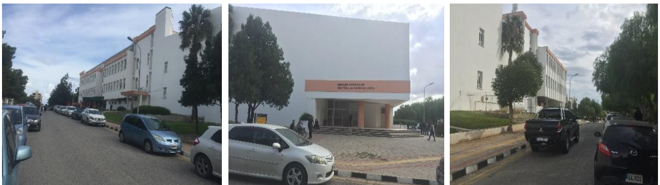
Fig 12: View showing set-back from Major Road, Main Entrance and Minor Road
